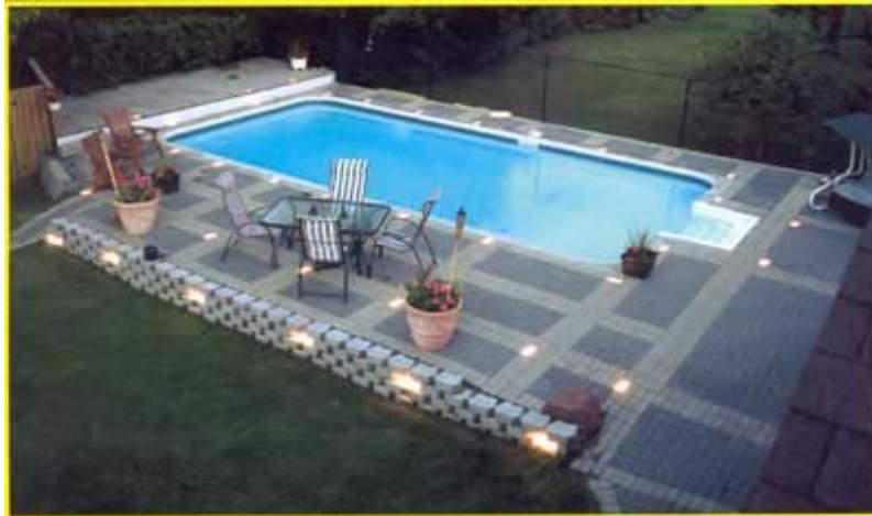
Pool with 4"x8" pavers installed in deck
