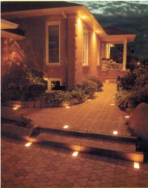
Sidewalk with 4"x8" pavers
