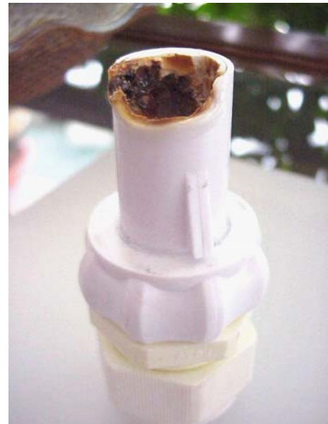
This one was not
