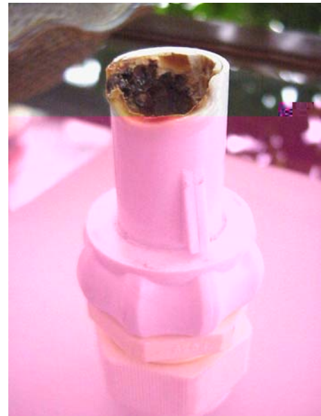
This one was not
